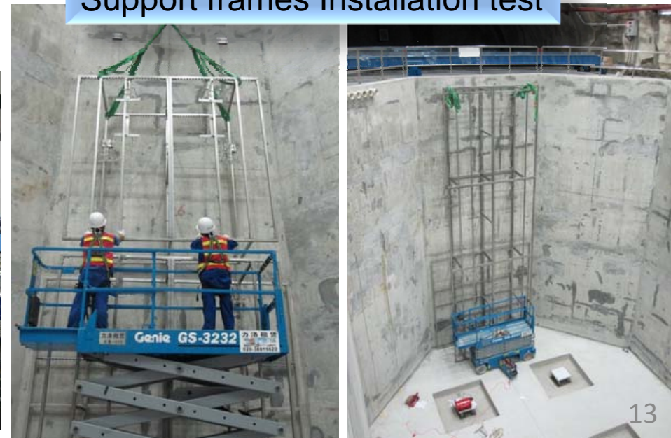
Support frames Installation test
