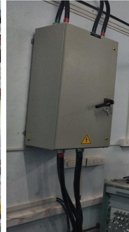
Polarity reversal switch for demagnetization
